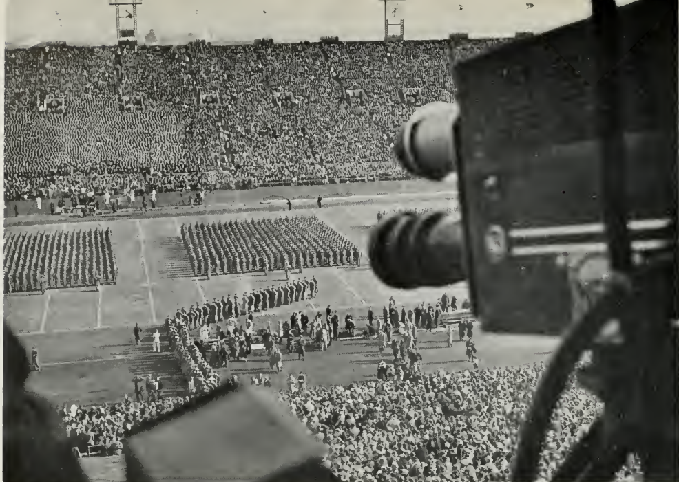
HIGH ON THE STADIUM ROOF, AN NBC TELEVISION CAMERA CATCHES THE FORMATION OF WEST POINT CADETS PRIOR TO THE ARMY-NAVY FOOTBALL GAME AT PHILADELPHIA. PICTURES WERE TRANSMITTED TO WNET, NEW YORK, OVER AN 80-MILE COAXIAL CABLE.
